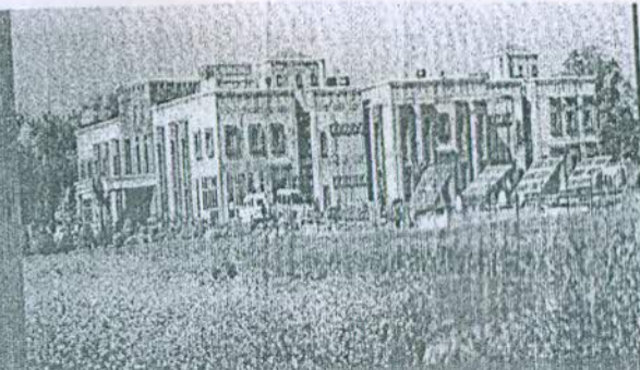
Administrative building cum Laboratory, ICAR- RCER, Patna
